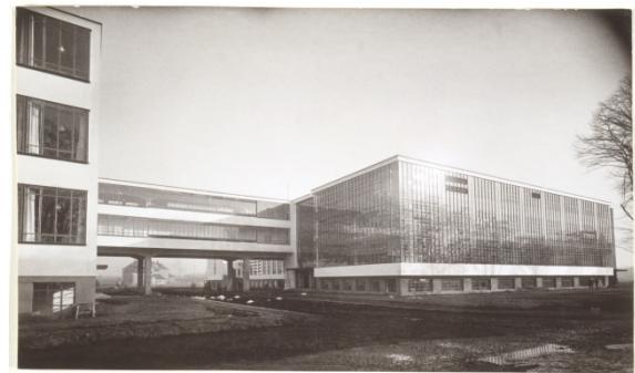
Lucia Moholy, Bauhaus building Dessau (architect Walter Gropius), 1926, Photo Credit: Bauhaus-Archiv Berlin © VG Bild-Kunst, Bonn
