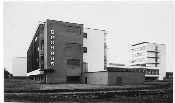
Lucia Moholy, Bauhaus building Dessau, view from the southwest with lettering, Architect: Walter Gropius, 1927, Bauhaus-Archiv Berlin © VG Bild-Kunst, Bonn 2026
